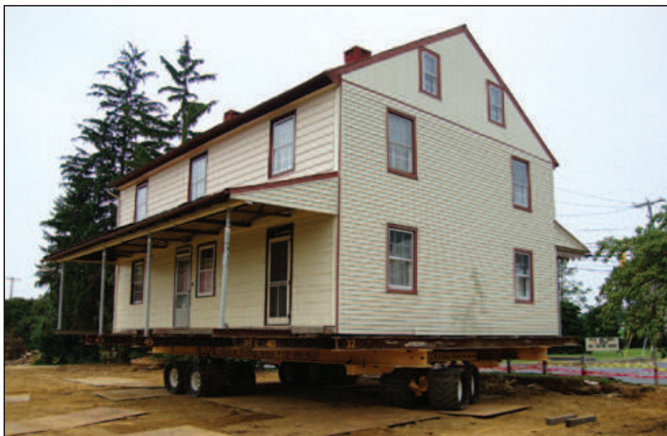
Figure 5R-1. House relocation (photo courtesy of Wolfe House Movers)
