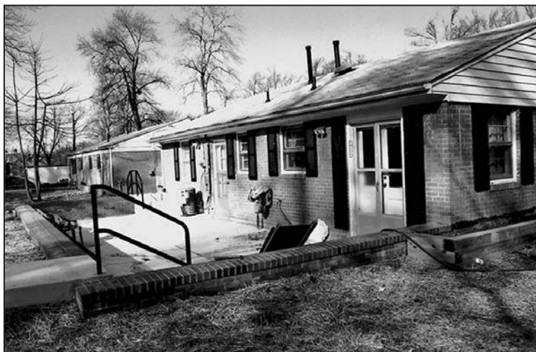
Figure 6-55. Brick-faced residential floodwall and access stairs
