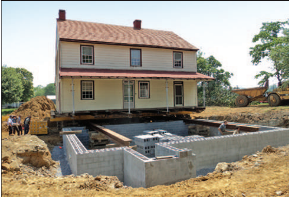
Figure 5R-10. New foundation wall construction begins (photo courtesy of Wolfe House Movers)
