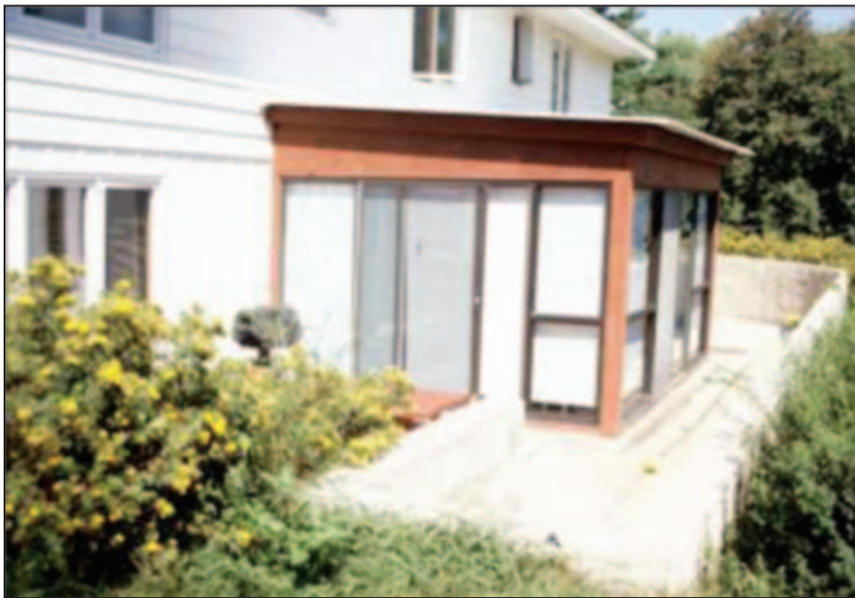
Figure 5F-2. Typical residential floodwall
