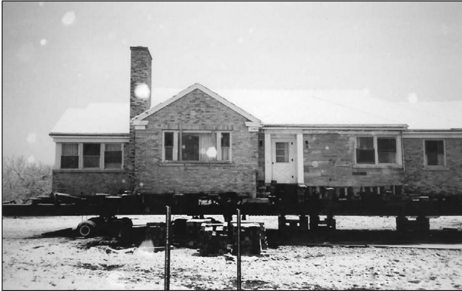
Figure 1-7. Structure placed on a wheeled vehicle for relocation to a new site
