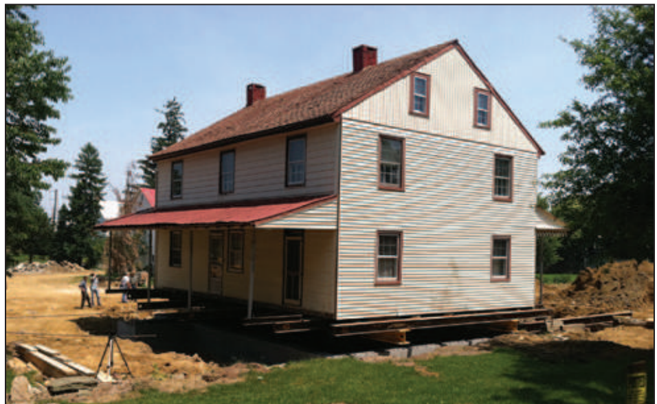
Figure 5R-13. House is lowered and connected to the foundation after foundation walls are completed (photo courtesy of Wolfe House Movers)
