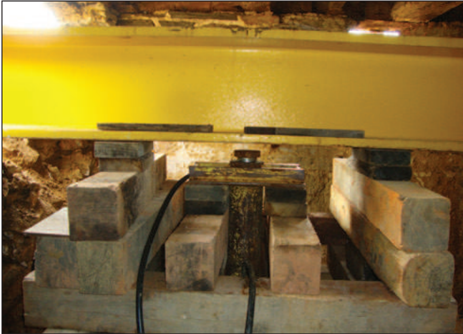
Figure 5R-7. Hydraulic jacks installed to lift structure from foundation (photo courtesy of Wolfe House Movers)
