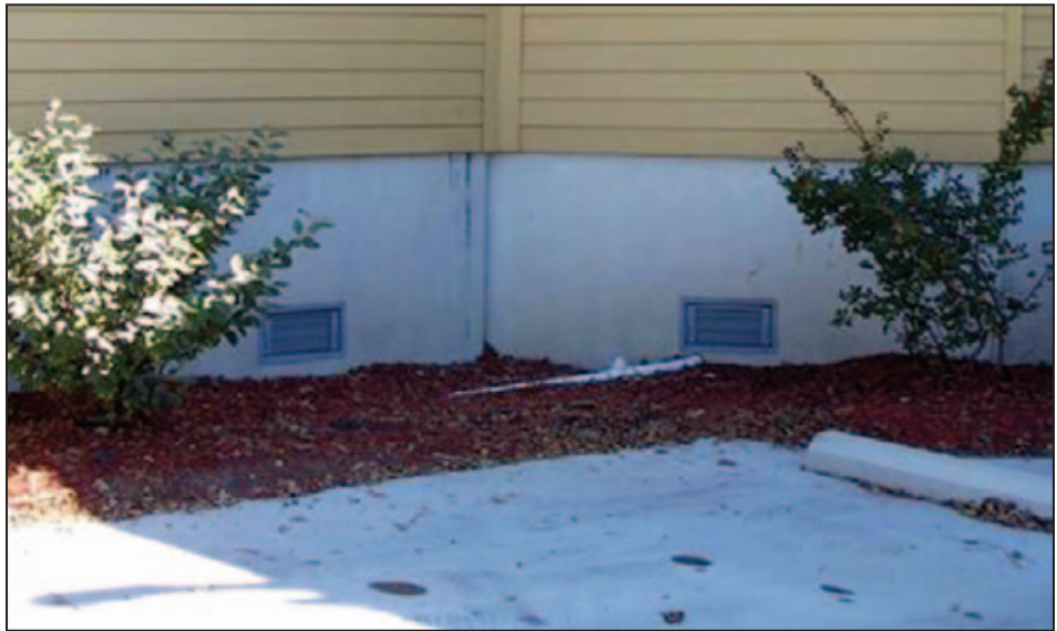
Figure 6-42. Example of flood vents
